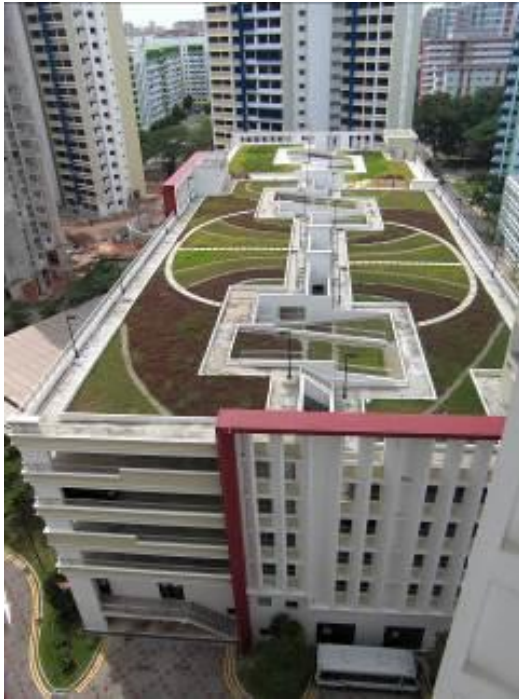
Fig. 2 Singapore-Tah Ching Jurong.JPG. Singapore has started a very ambitious programme to support sky-rise greenery, Courtesy: IGRA.
