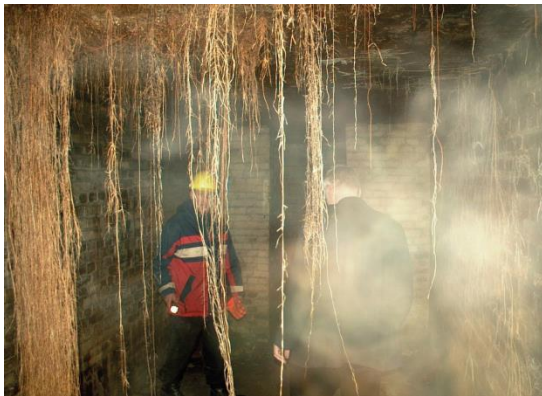
Fig. 1 Root threads in war bunkers. (City of Osnabrück)
