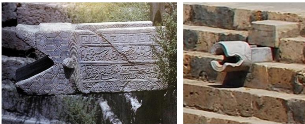
Fig.4 Using the symbolic element of “lion head” as the water entrances to the pools. Source: Timur & Mankovskaja, 1991
