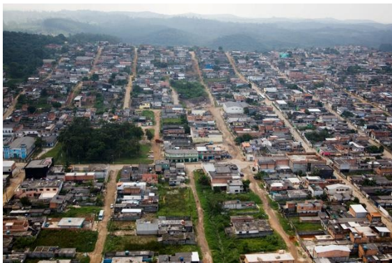
Fig.1 Vargem Grande, São Paulo - Housing Programme, general view.
