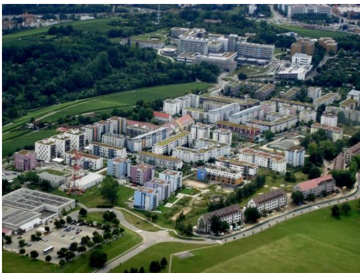
Fig. 1 GRA-Stuttgart.jpg. The aerial view demonstrates the success of the Green Roof policy in Stuttgart, Courtesy: IGRA.
