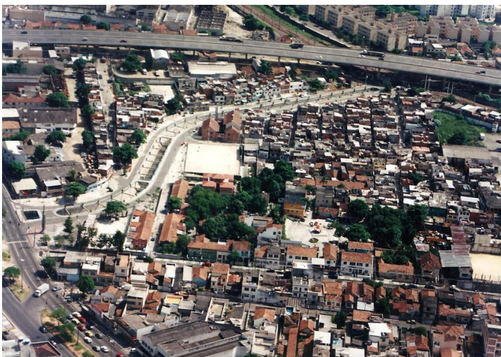
Fig. 3. Second urban projects’ generation: Programa Favela Bairro (Favela-Neighbourhood Programme) at Favela Fernão Cardim, in Rio de Janeiro’s suburban area. Source: Jorge Mario Jáuregui @telier Metropolitano ( www.jauregui.arq.br/ ).
