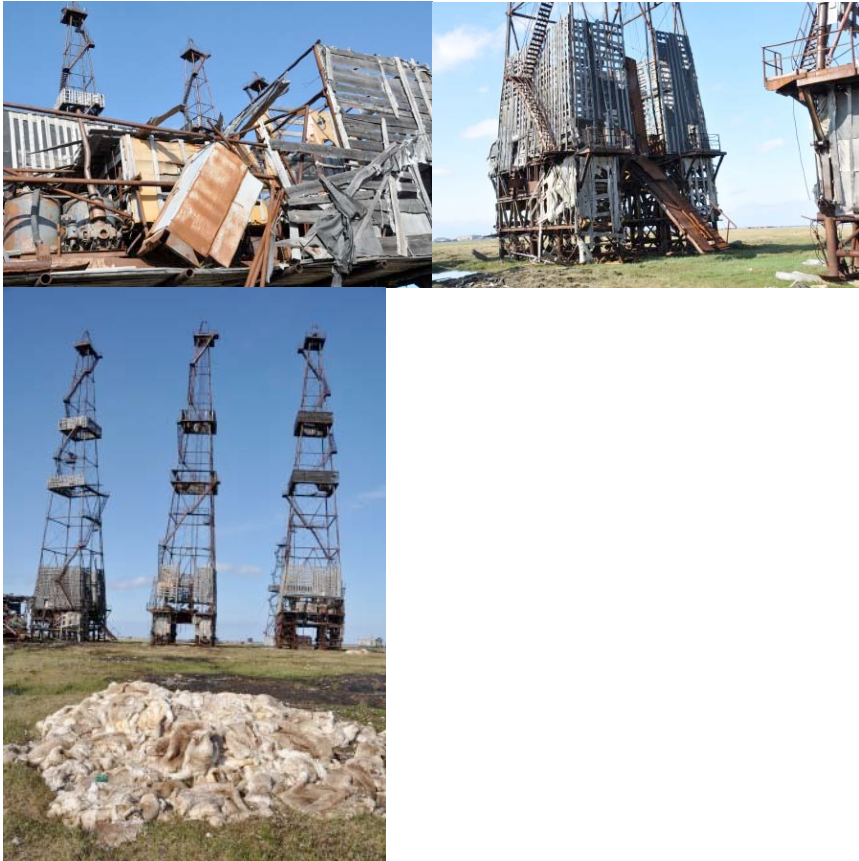
Debris from drilling rigs and associated buildings. Lower photo shows one of 15 piles of reindeer hides scattered about the tundra near the drilling rigs.
