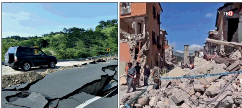
Fig. 5. Destruction caused by earthquakes with M = 4.2 . Left – Veliko Tarnovo, Bulgaria. Right – Norcia, Umbria, Italy; Sources: https://pronedra.ru/uploads/d/cP/OC/cPOC-mQu3.orig.jpg and http://www.tvc.ru/news/show/id/99704#&gid=1&pid=2 .
