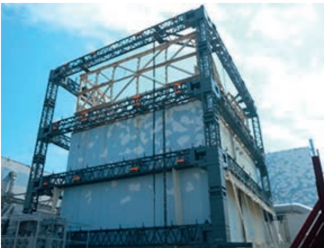
FIG. 7. Reactor cover construction at Fukushima Daiichi Unit 1. Photograph courtesy of the Tokyo Electric Power Company (TEPCO) [24].
