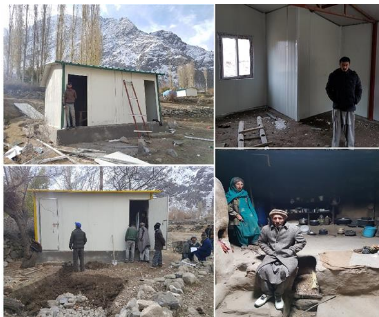
Fig. 10. Shelters under construction. Photographs credit: AKAH Pakistan
