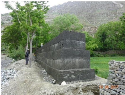
Fig. 11. Cross-sectional view of protection wall along the gorge at the convex portion of the meandering stream
