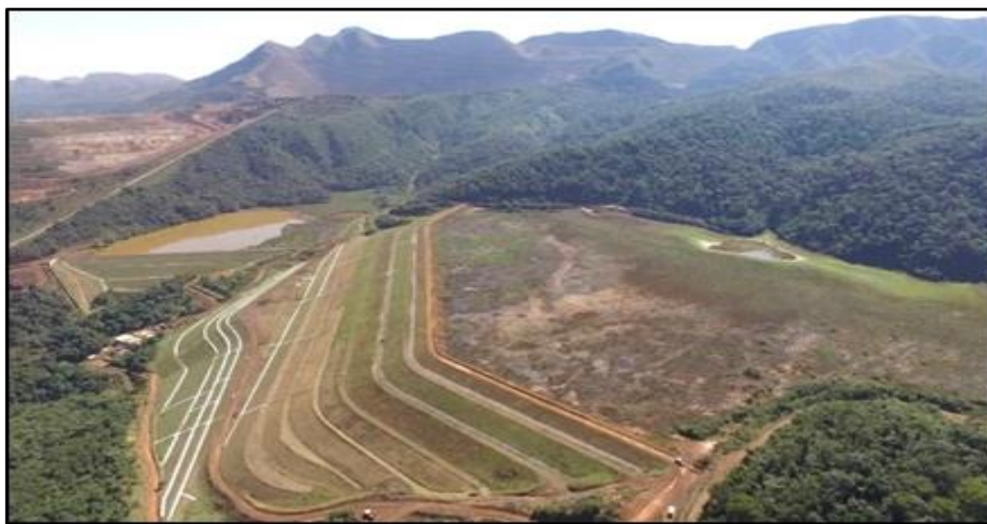
Fig. 2. Brumadinho Dam and Reservoir before rupture with the undrained water puddles on its surface
