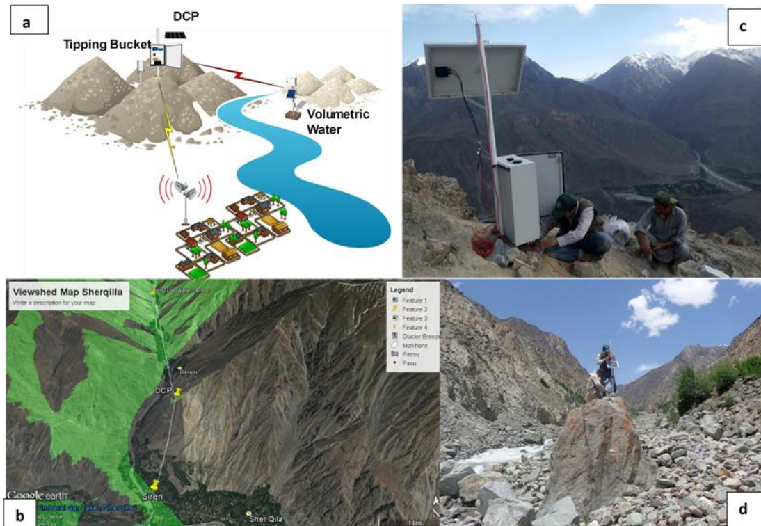
Fig. 6. a) Describes the early warning system and its components i.e. water content sensor, data collection platform, tipping bucket and siren system. b) Selection of site through the remote sensing to view the line of site for EWS. c) AKAH staff installing DCP at the identified site. d) Installation of water content by staff. Photo Credit AKAH Pakistan
