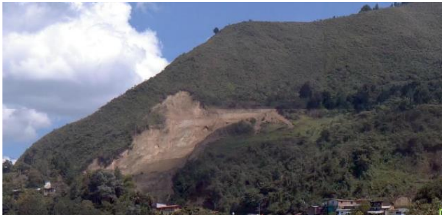
Fig. 24. Remediation works on March 2017
