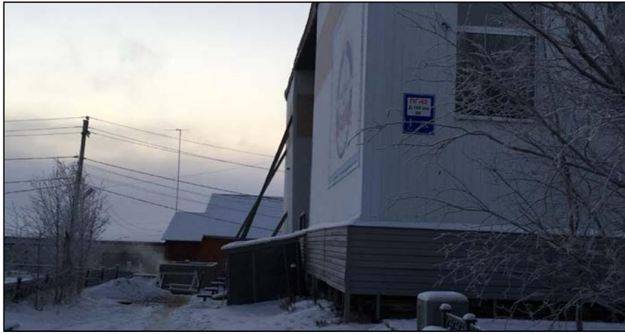
**Figure 1:** Differential Settlement of the Building of Yamal Polar Agricultural College
