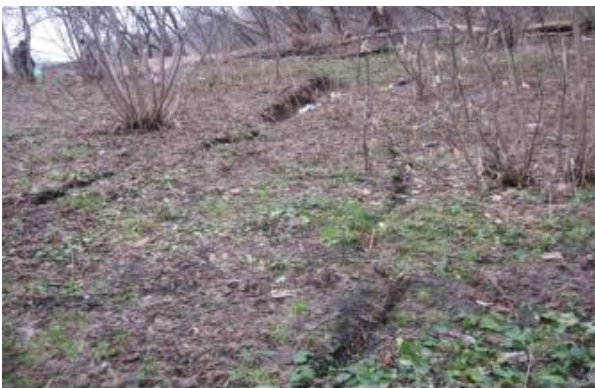
Figure 5 Sliding fracture of lower sliding blocks opposite the temple
