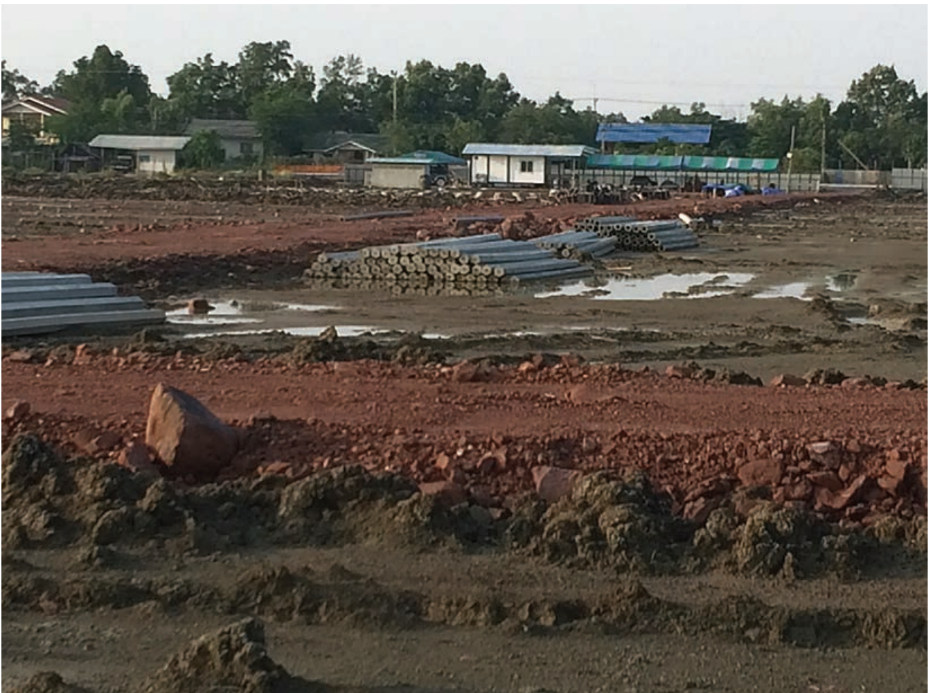
Construction works at Khok Kham, Sep 2016
